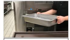
Empty drain pan each time the water level reaches half full.
